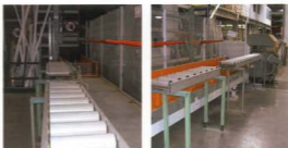
Tashman's safety nightmares ended when he installed a Kasto automatic storage and retrieval system. The whole system is fenced and sensed throughout, and it will not operate when a person is inside the area.
